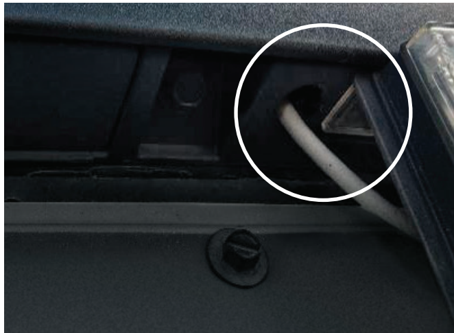
Close up of after-market light and wiring.
